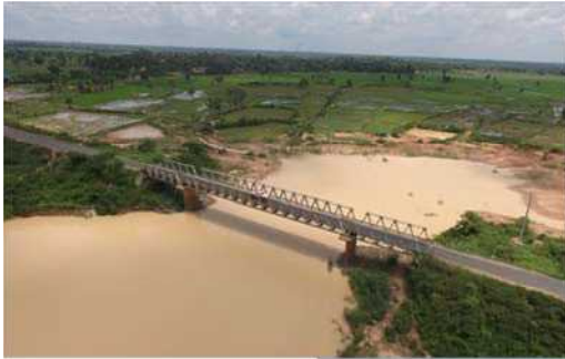
Ba Baong 2 Bridge on NR11
